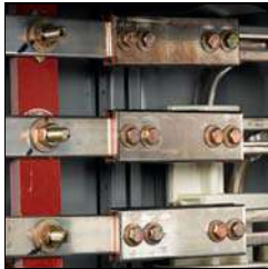
Horizontal Bus Splice
