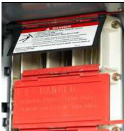
Automatic Vertical Bus Shutter
